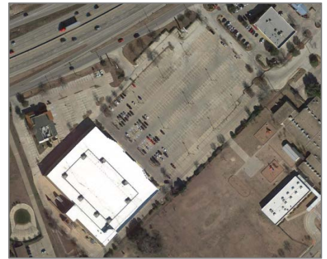
Figure 6.2: Kohl's Parking Lot, which recently was subdivided to incorporate a Cracker Barrel restaurant at the northeast corner.
