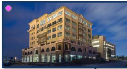
1 Trend Tower Office Building
