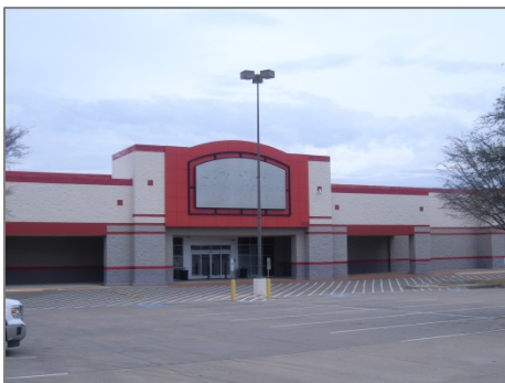
Figure 6.1: Vacant Sports Authority building prior to being converted to an Academy this year.
