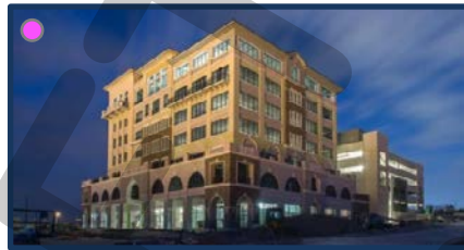
1 Trend Tower Office Building
